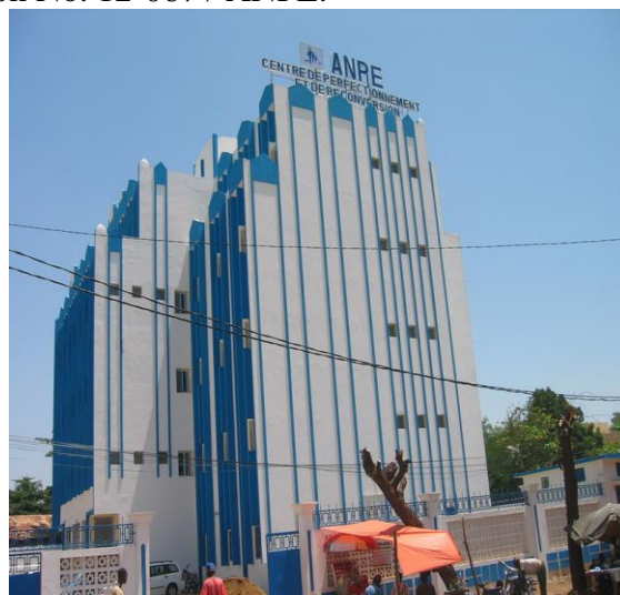
The building housing the CPR/ANPE in Bamako
